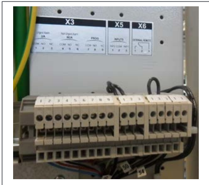
Figure 24. Alarm dry contacts
