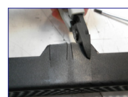
Cut holes to allow cable access
